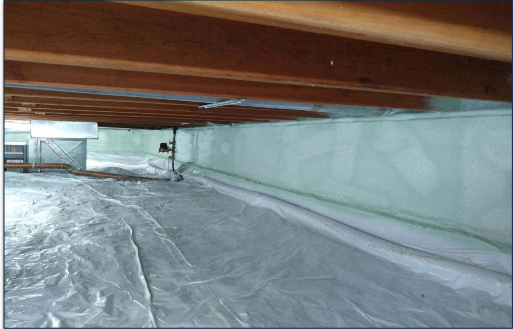
Radon Mitigation/Crawl Space Insulation
