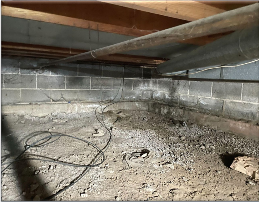
Dirt Floor Crawl Space
