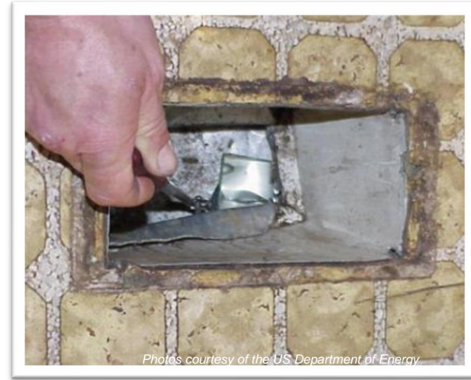
Check the flanges and inspect for damage
