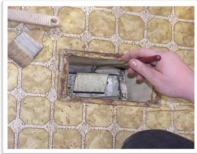
Inspect for blockage and loose seams
