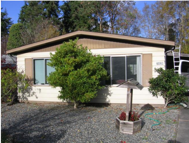
Open Attic Cavity
