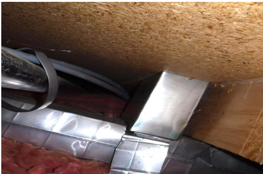
Riser crosswise joists
